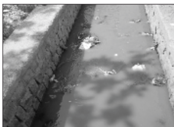
Picture 5: Bapu Nagar-Storm Water Drainage
