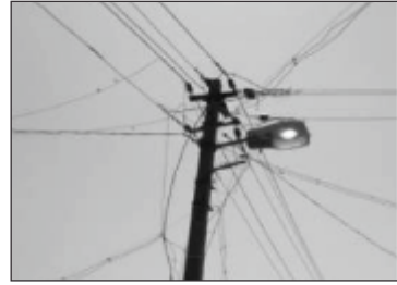
Picture 10: Mangarwadi -Street lighting
