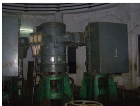
Deteriorated Conditions of Pumps
