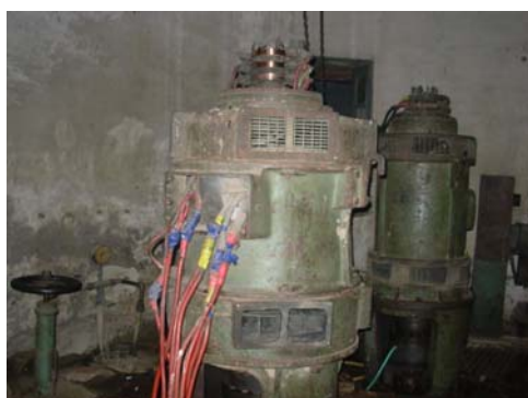
Deteriorated Conditions of Pumps
